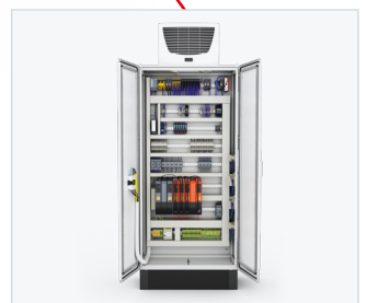
The control electronics, safety engineering and industrial PC are installed in the control cabinet .
